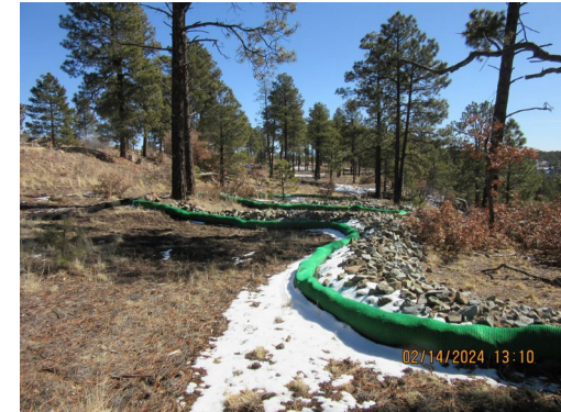
Compost logs (2024) and rock check dams (2015)
