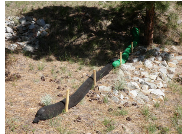
Coir log (2024), rock check dam and plunge pool (2019)
