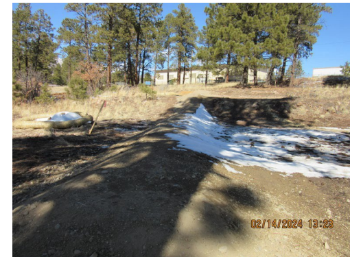
Base course berm (2024)
